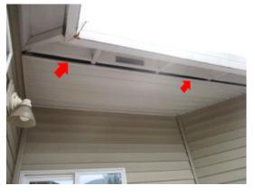
The siding on the front garage side walls was cut too short to fit properly in the J-channels. The siding was screwed to the wall. Vinyl and/or Metal siding should not have any fasteners secured through the siding.
