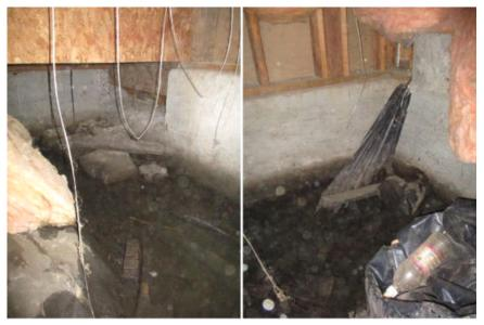
There is also a low area under the Western half of the living room area. It would be recommended to trench from this low area to the kitchen low area to allow drainage. It would be recommended to install a crawlspace access door in the rear garage wall to more easily access the crawlspace. Additionally a sump pump would be recommended in this low area and an access near the sump location will make maintenance of the sump easier.
