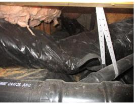
The furnace ducting is lying on the ground under the front office, in the crawlspace. The ducting should be raised up off of the ground and supported.
