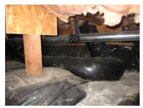
There is debris noted in the ends of a number of the ducts, near the floor registers, around the crawlspace. This was noted by knocking on the ducting and feeling or hearing debris inside of the ducting. It would be recommended to have the ducting cleaned or vacuumed to remove any and all debris.
