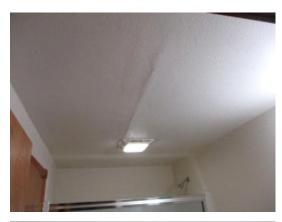
There is a very large patch in the living room ceiling. It is suspected there may have been a past leak from the upper bathroom. No leaking was noted at the time of the inspection.
