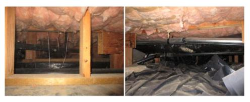
There is standing water in the crawlspace under the kitchen, at the rear garage foundation wall. It would be recommended to install a crawlspace access door in the rear garage wall to more easily access the crawlspace. Additionally a sump pump would be recommended in this low area and an access near the sump location will make maintenance of the sump easier.
