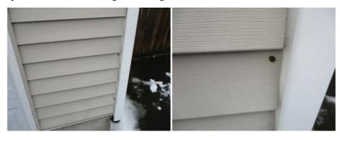
There are several holes and punctures through the siding. The damaged sections of siding should be replaced or properly patched.
